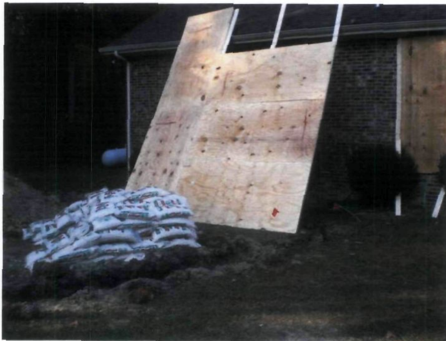
Figure C-18: Engineering Controls for 81 MM Mortar, Area 4C - 4542D Uzzle Road
